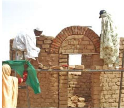
**Pic 9.** The door arch using method 2; a girder made from bricks and muna
